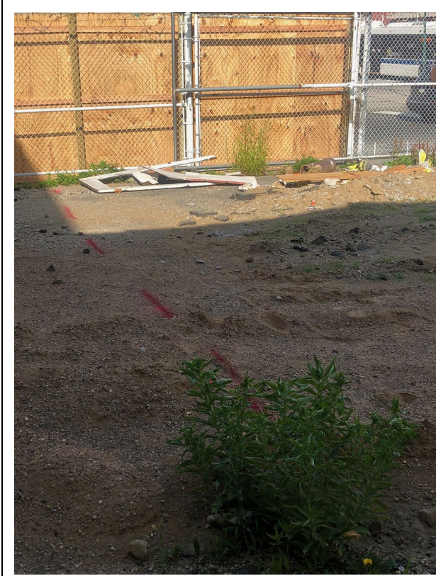
Fig. 1: Old Electric Feed from street
