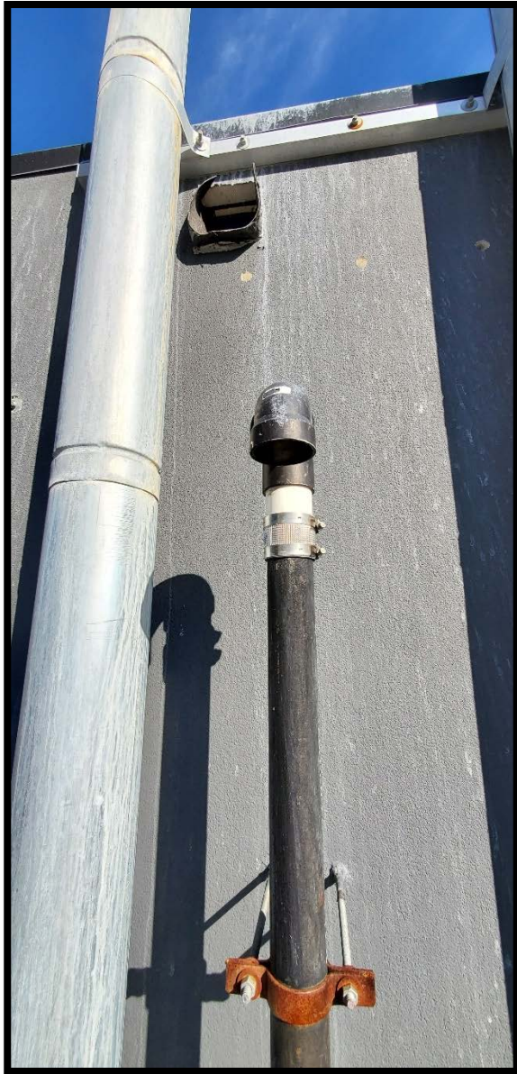
View of the SSDS discharge on the roof.
