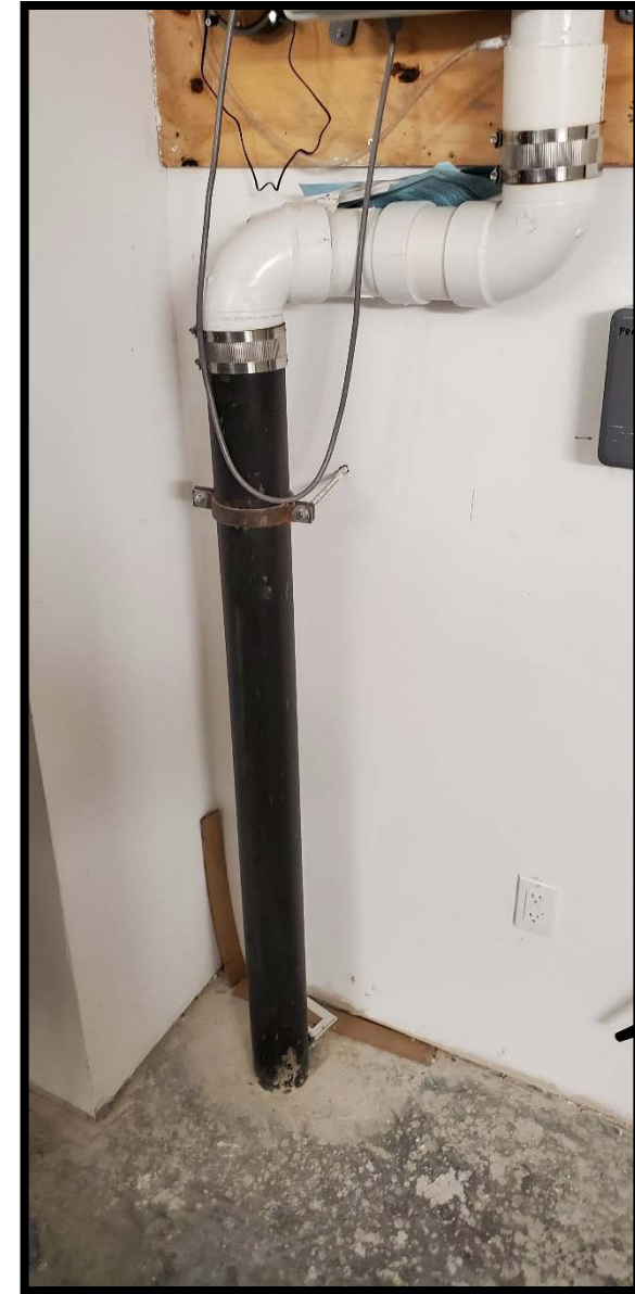
View of the SSDS riser pipe.
