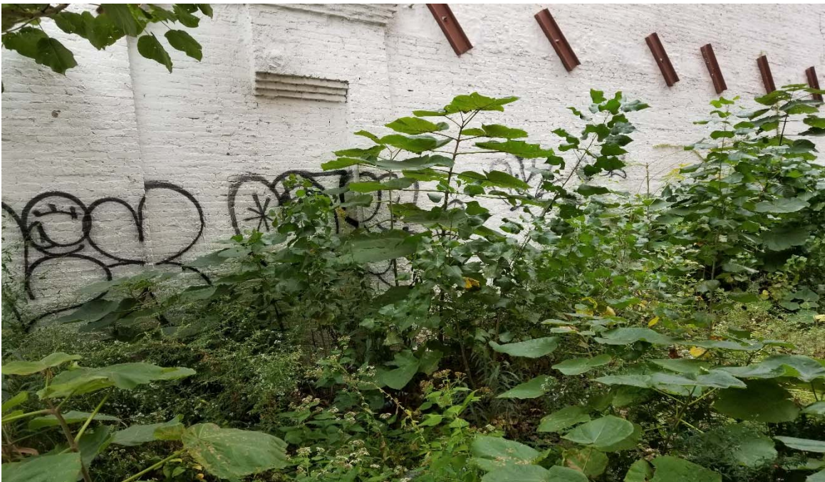
View of Site, looking south.
