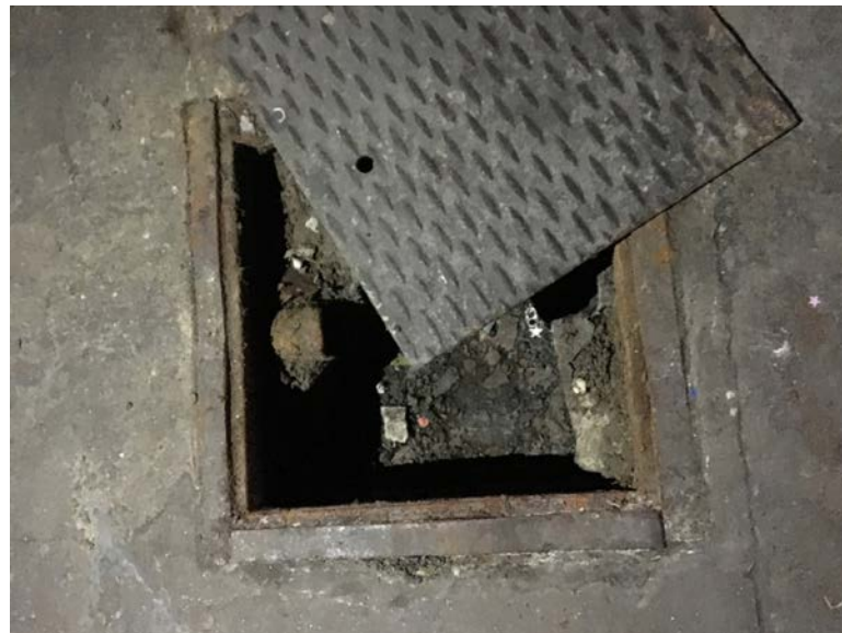
View of drain pit with soil
