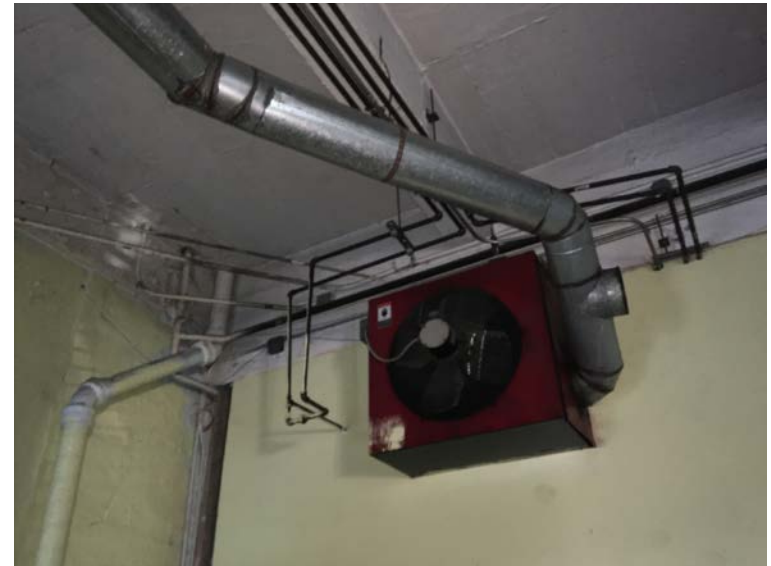
Wall mounted fan- heating
