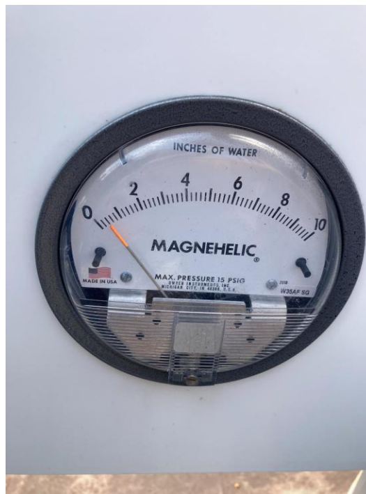
Photo 6: View of the magnehelic gauge on the SMD roof exhaust system (facing south). Taken 7/25/2023.
