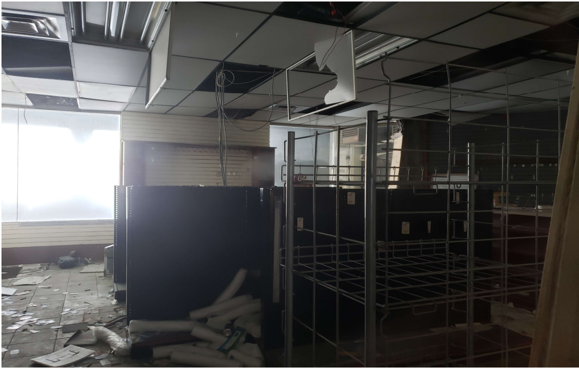
View of Site building interior, including suspect ACM containing ceiling tiles and suspect PCB-containing fluorescent light ballasts.
