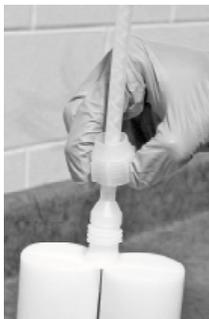
\* The ports can be removed by striking with a hammer after foaming is complete in about 3 or 4 hours. Grind off the surface seal epoxy for a smooth finish. The surface seal epoxy is paintable if desired.
