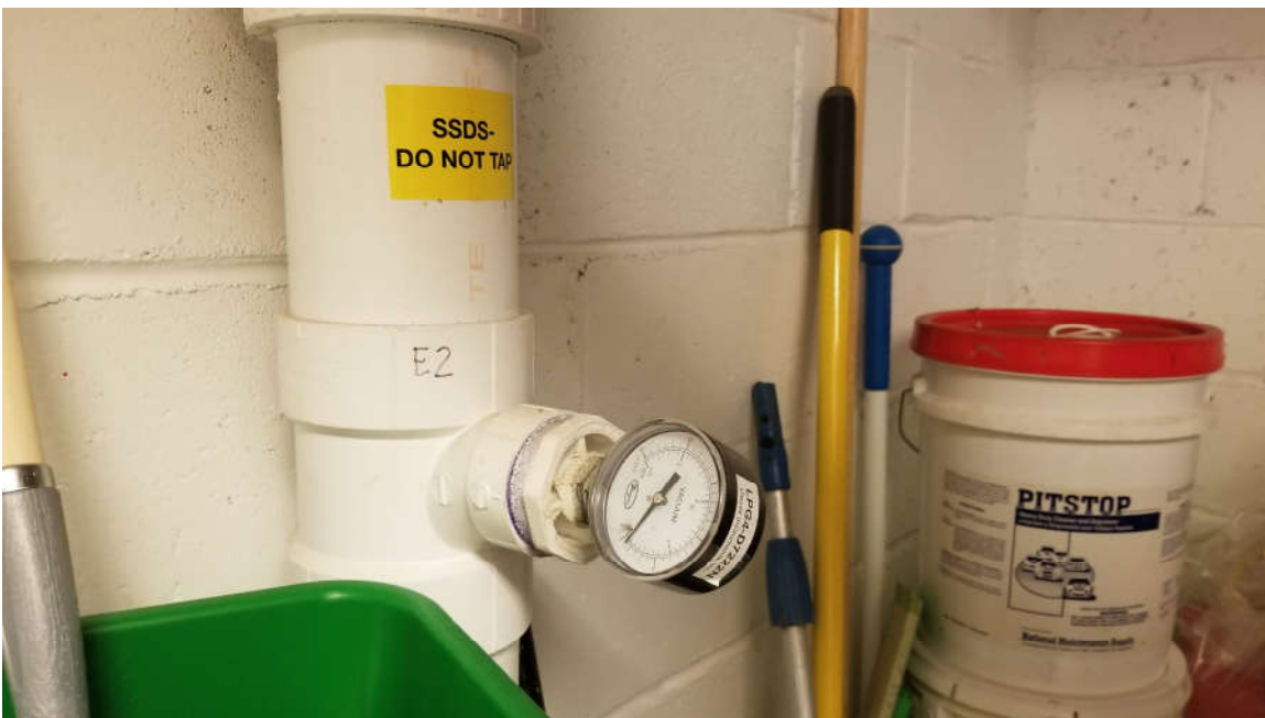
Photo 12: SSDS air conveyance piping and control valve at riser E2.
