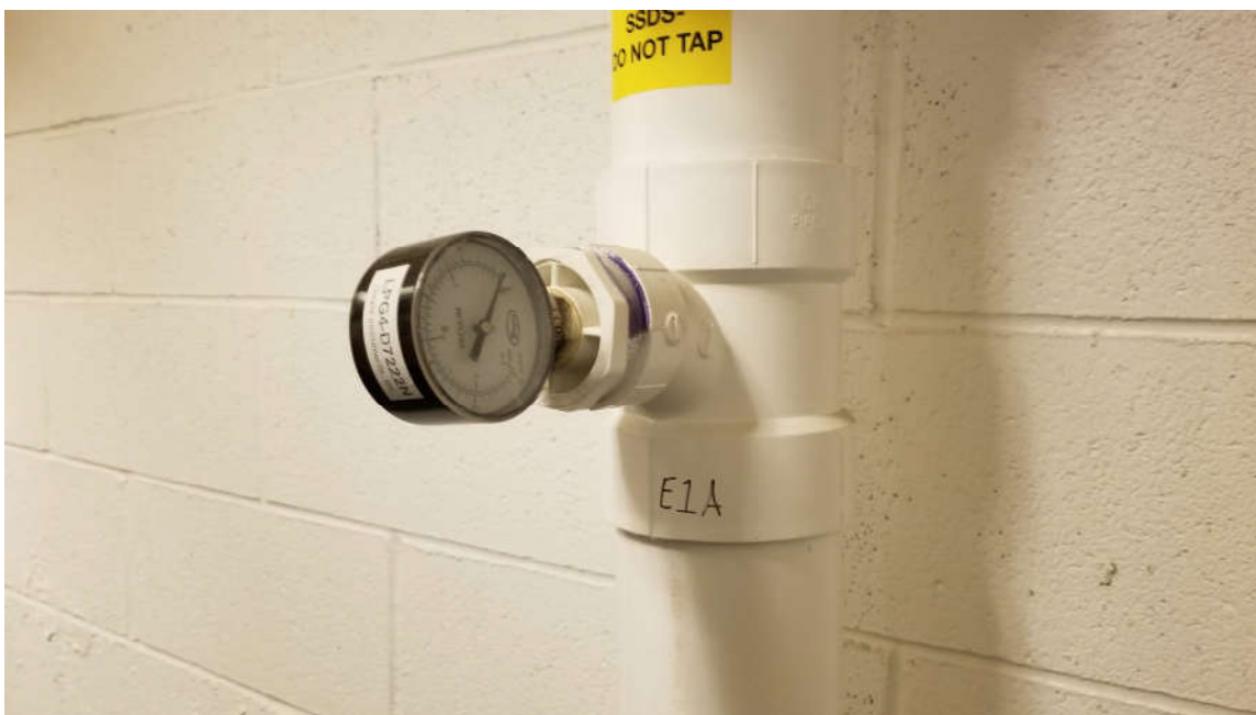
Photo 14: SSDS air conveyance piping and vacuum gauge at riser E1A.
