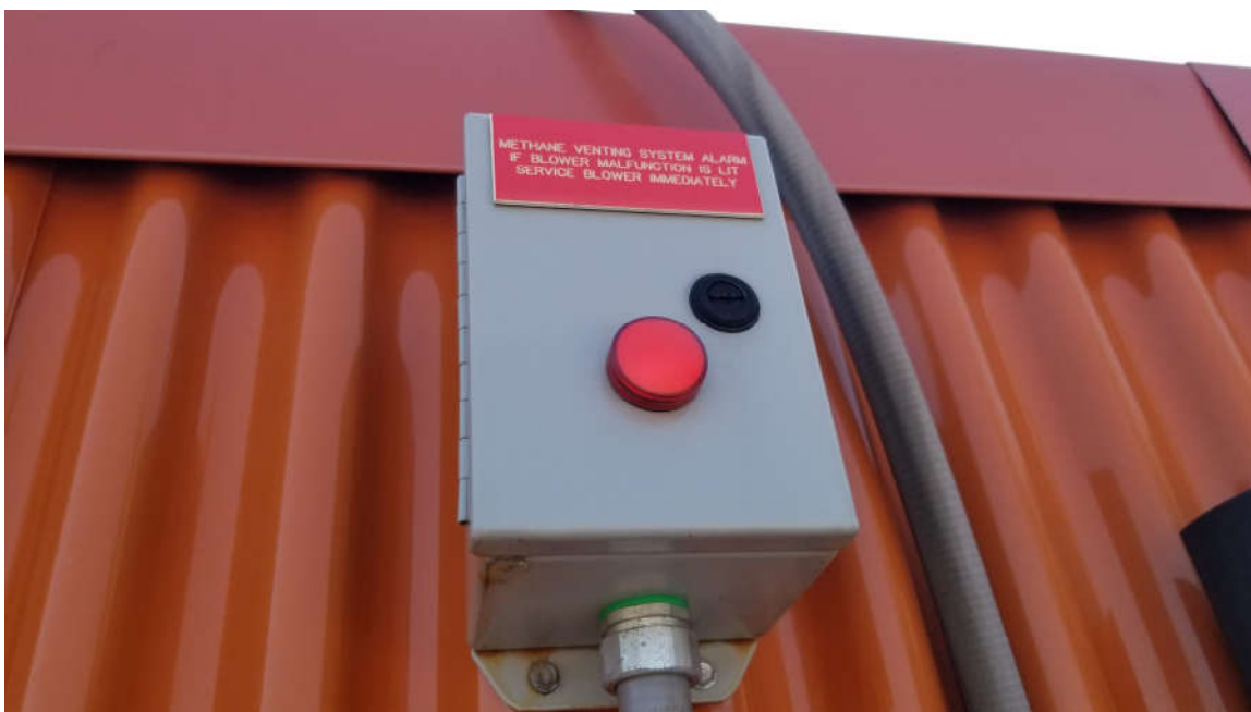
Photo 15: View of SSDS alarm panel.
