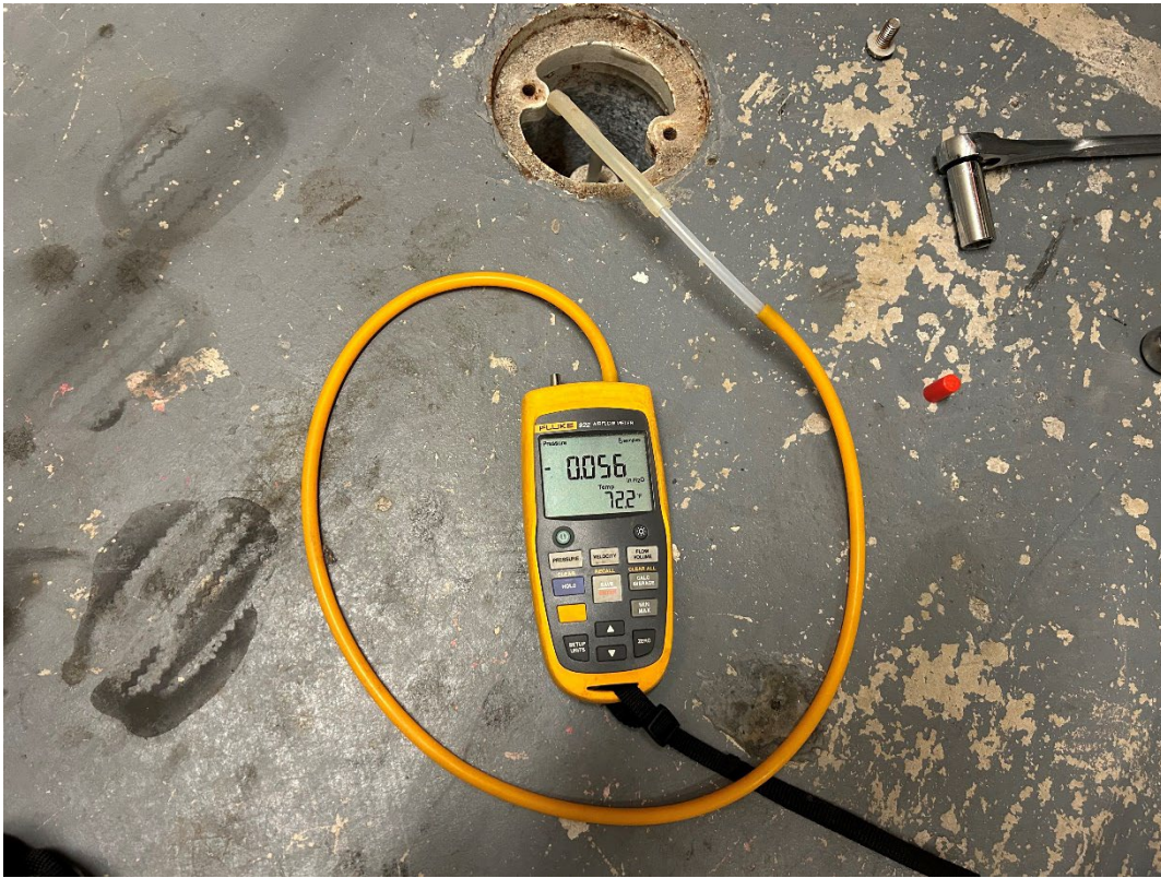
Photograph 13: View of the micromanometer measurement at the SSDS monitoring point SV-1.
