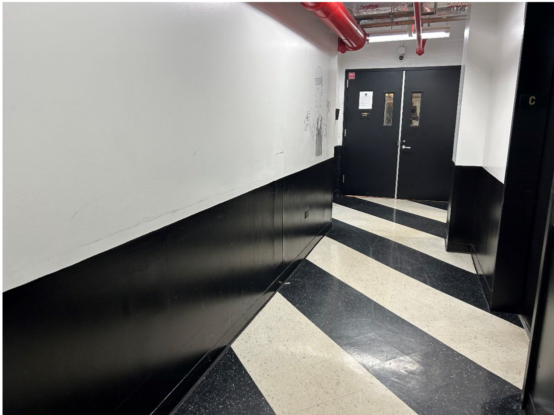
Photograph 2: View of the basement walls and flooring.
