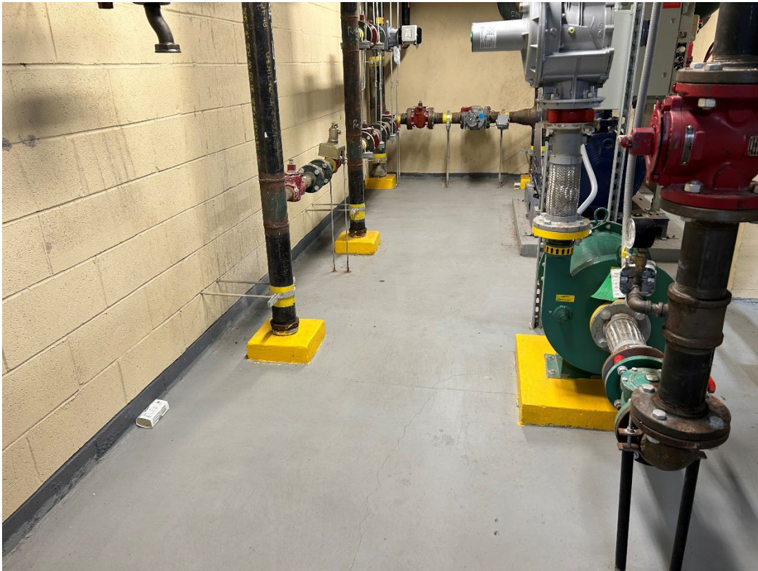
Photograph 1: View of the basement floor.
