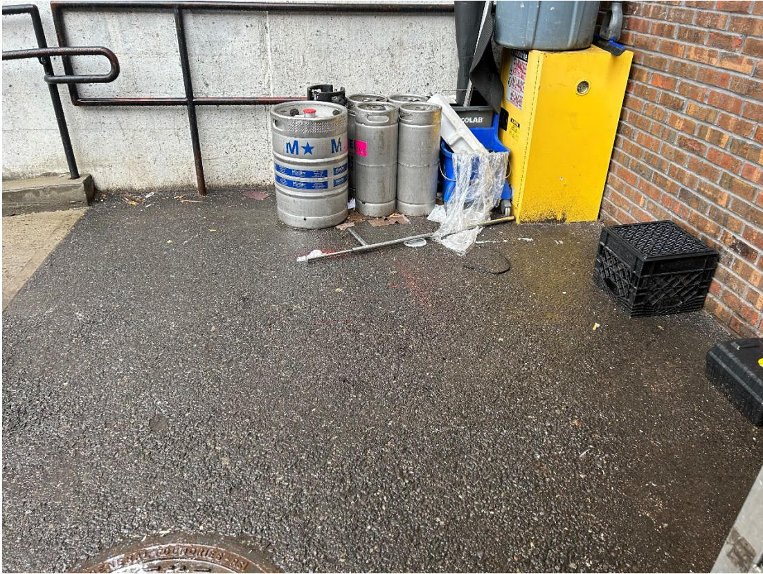
Photograph 9: View of the asphalt cover in Lot 42.
