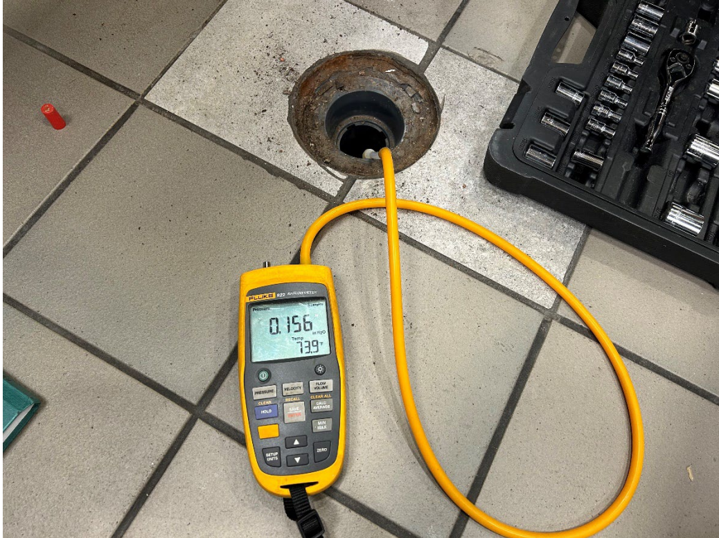
Photograph 14: View of the micromanometer measurement at the SSDS monitoring point SV-2.
