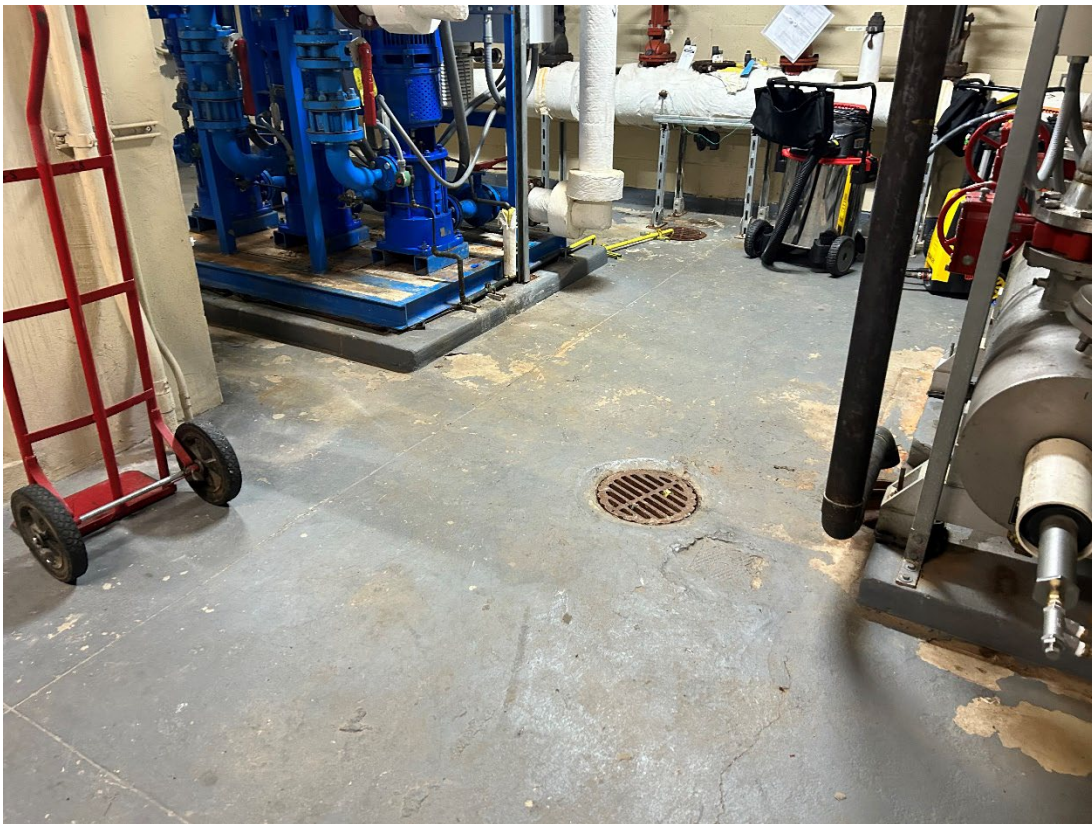
Photograph 4: View of the basement slab in a room with floor drains.
