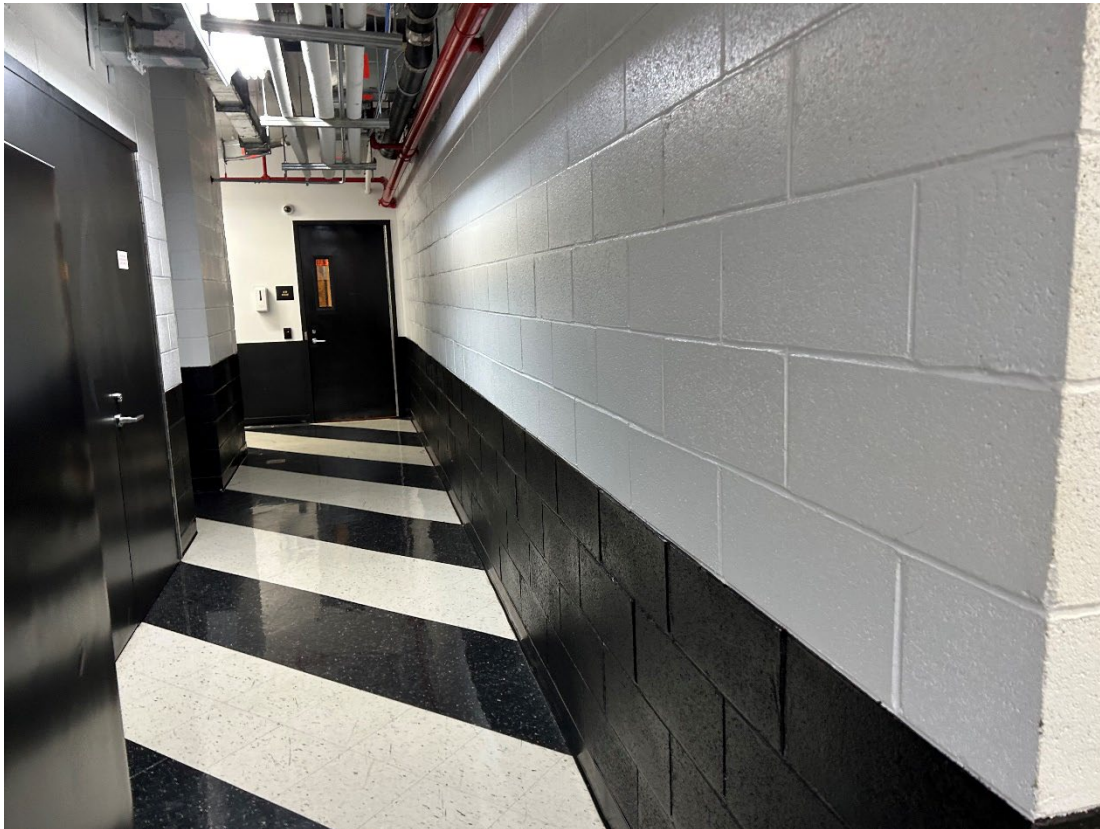
Photograph 5: View of the basement walls and flooring.
