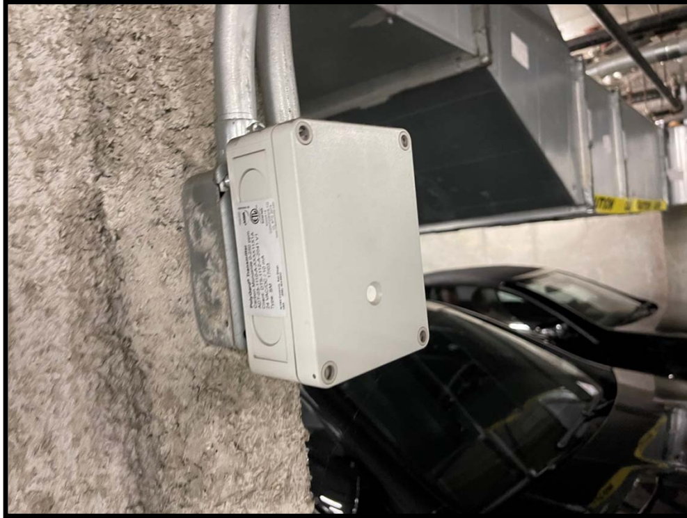
View of the ventilated parking garage alarm unit.
