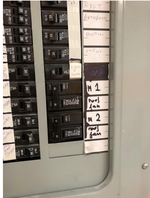
Labeled Circuit Breakers
