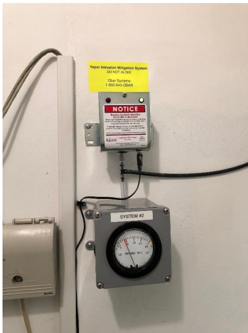
System Alarm and Vacuum Gauge
