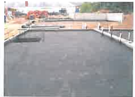
ULTRASHIELD™ G-1000 is a needle-punched non-woven geotextile with superior tensile strength and puncture resistance.
