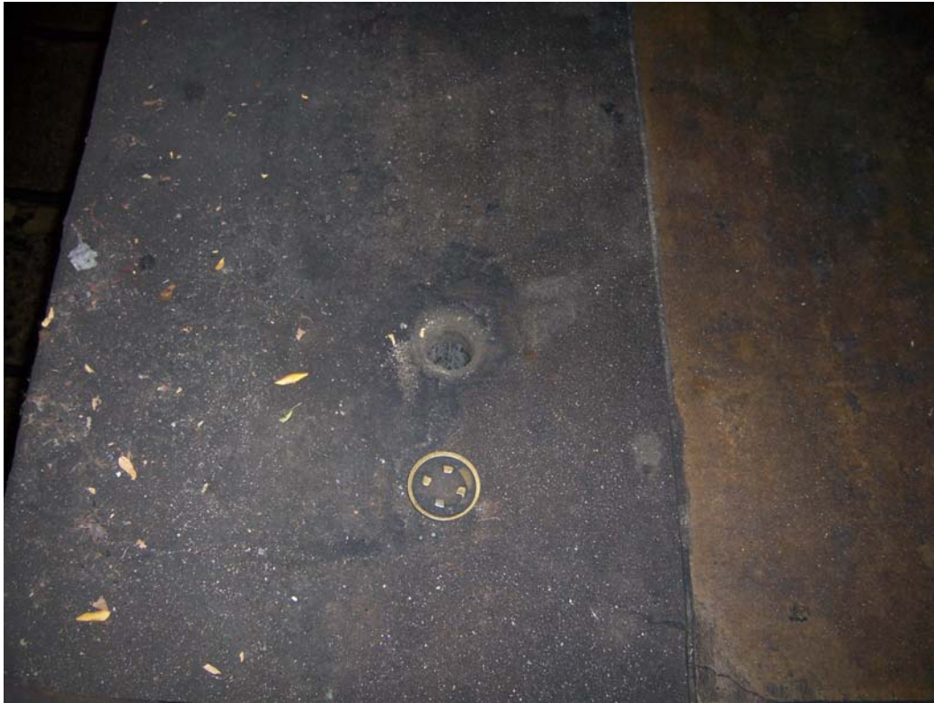
Photo 7: View of oil fill port located on the second floor associated with 550-gallon AST on the first floor.
