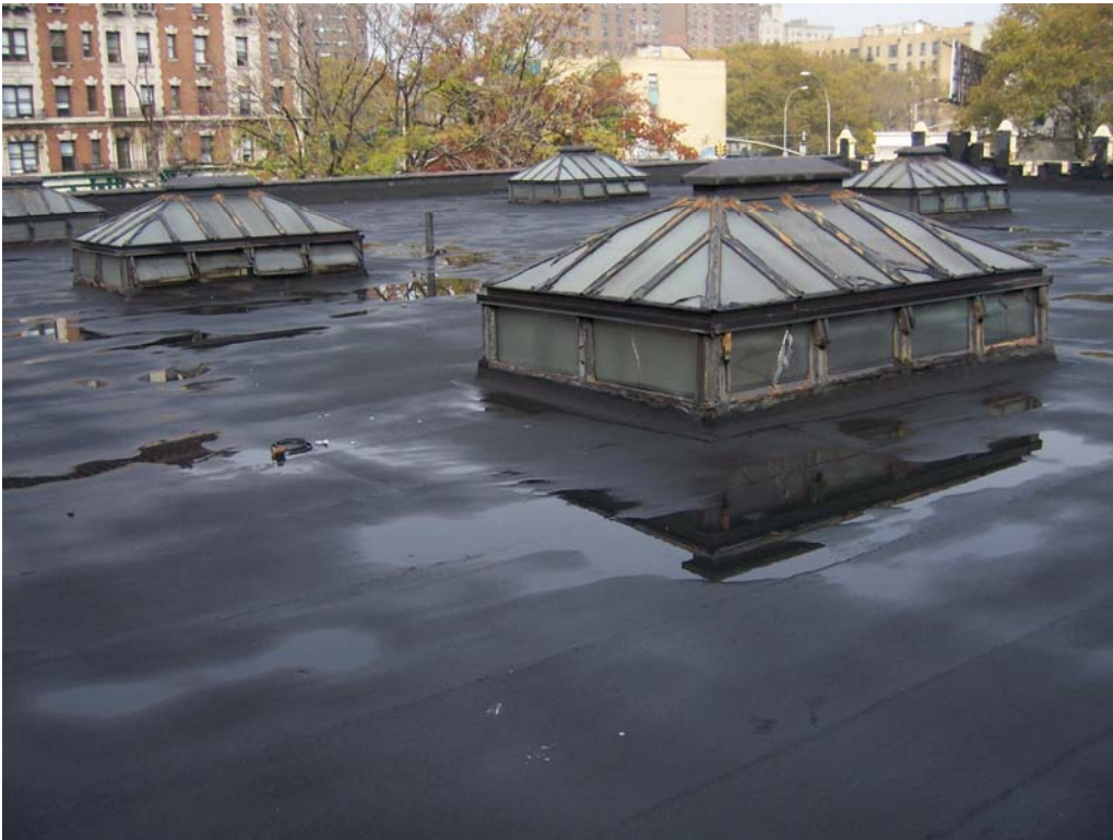
Photo 6: View of roof.
