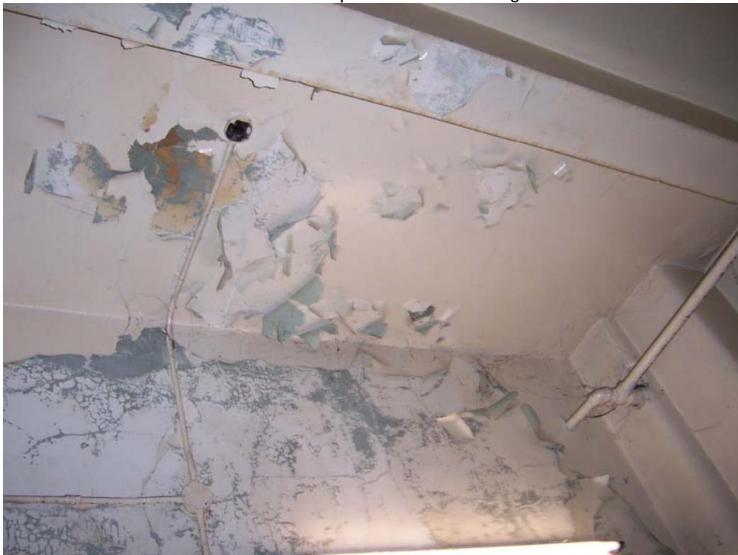
Photo 10: View of excessive peeling paint in the bathroom next to the office on the first floor.
