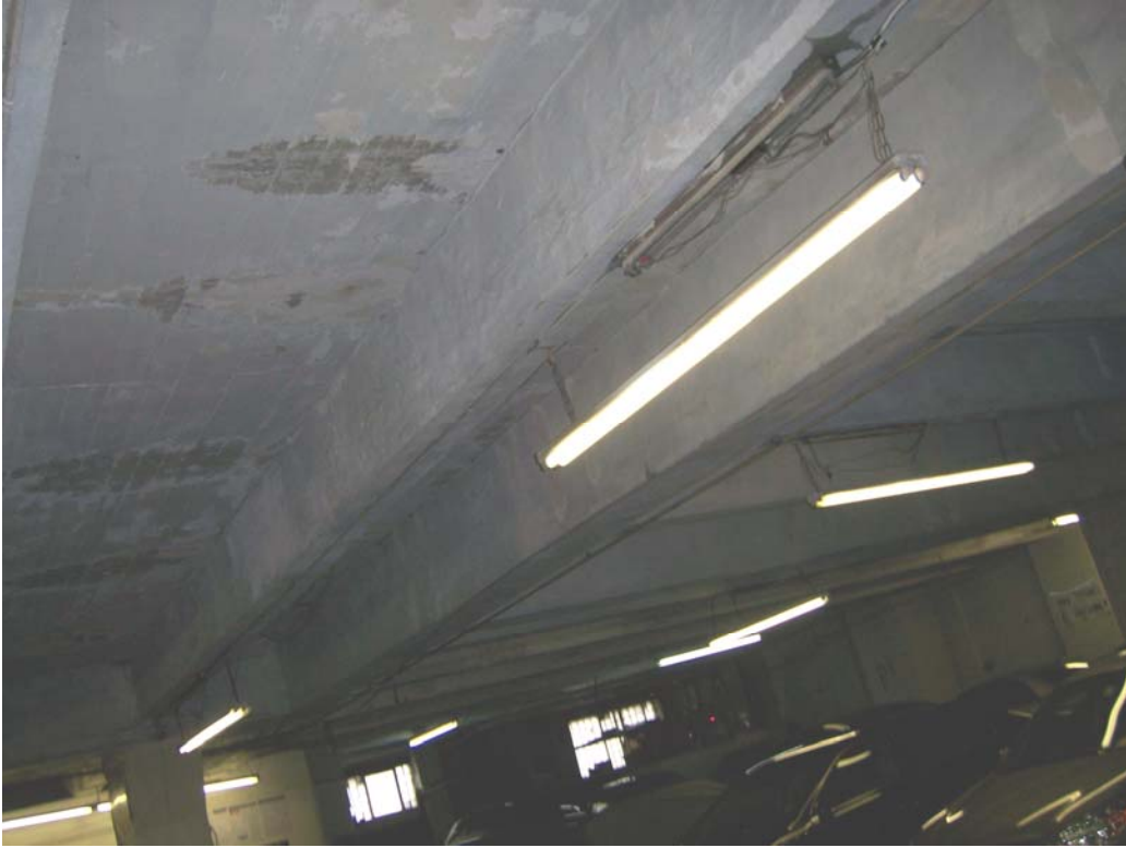
Photo 3: View of typical ceiling.
