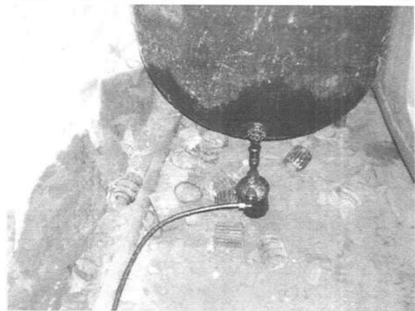
14. View of the dirt floor beneath the AST.
