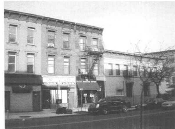
24. View of the adjacent mixed-use building to the east (facing north).
