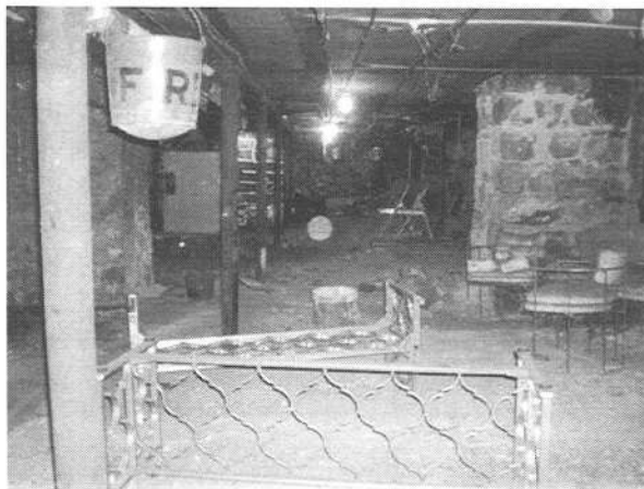
15. View of the eastern basement area.
