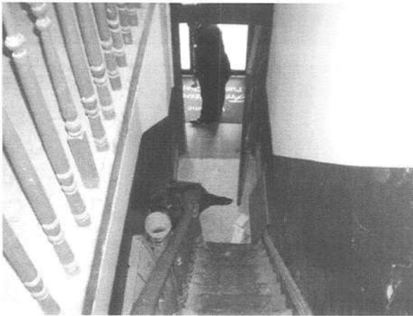
21. View of stairway leading to apartments.
