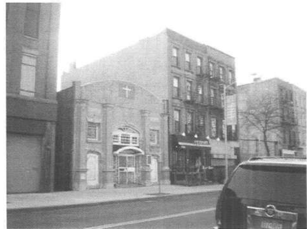
22. View of the church and commercial/residential buildings to the south across Fulton Street (facing southwest).
