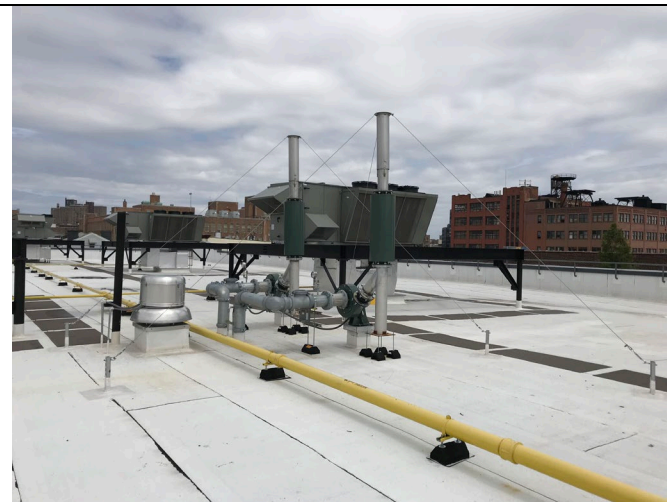
Photo 2: Inspection of SSDS fans, SF-2 and SF-3, and associated rooftop SSDS accessories.
