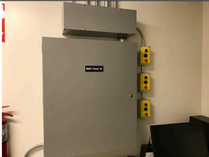
Photo 5: Inspection of alarm indication stations for SSDS.
