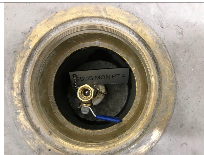
Photo 4: Inspection of interior of SSDS monitoring point, MP-4.
