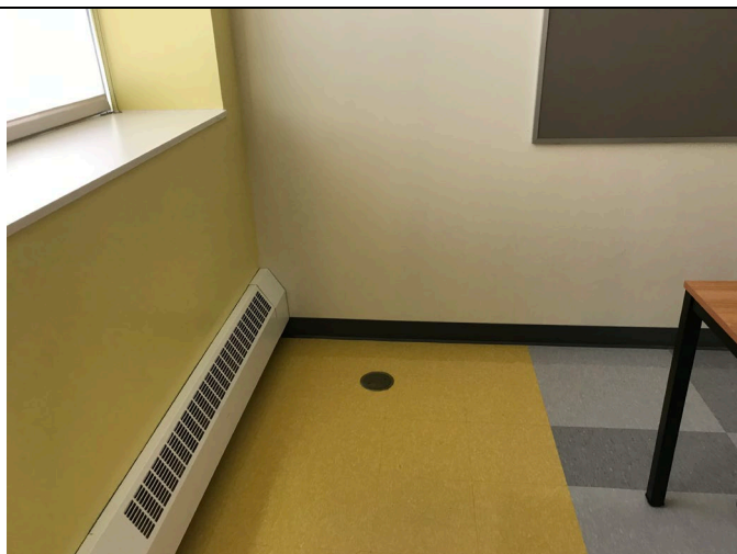
Photo 3: Inspection of SSDS monitoring point, MP-5.
