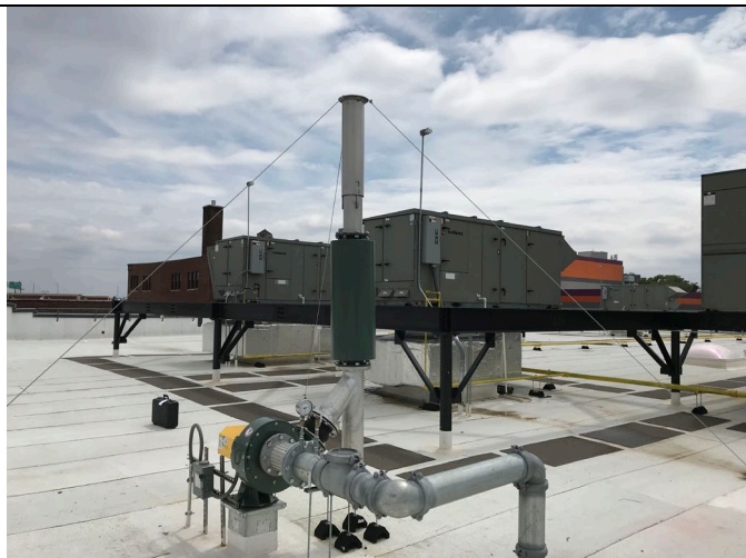
Photo 1: Inspection of SSDS fan, SF-1, and associated rooftop SSDS accessories.
