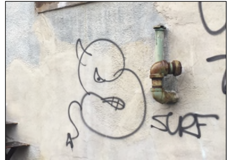
Photograph 12: Tank fill port and vent pipe located on the north-adjacent block.
