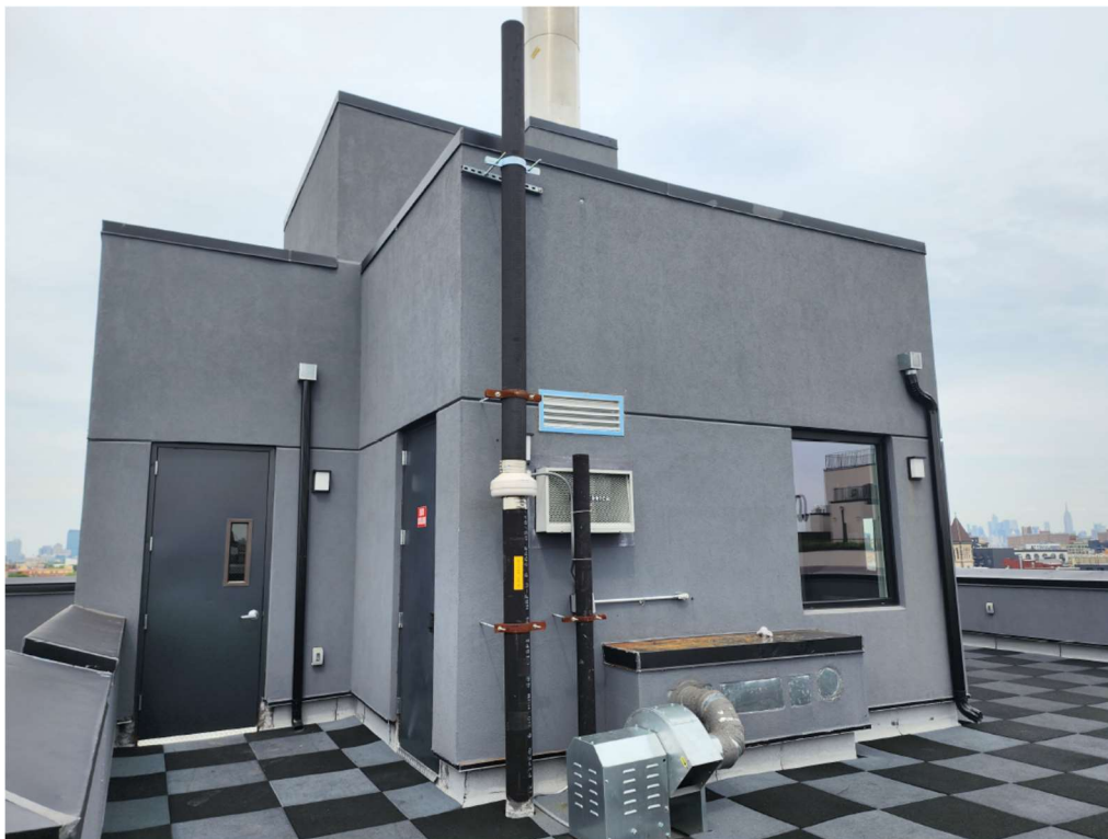
Photo 6 – View of the SSDS riser and fan on the roof.
