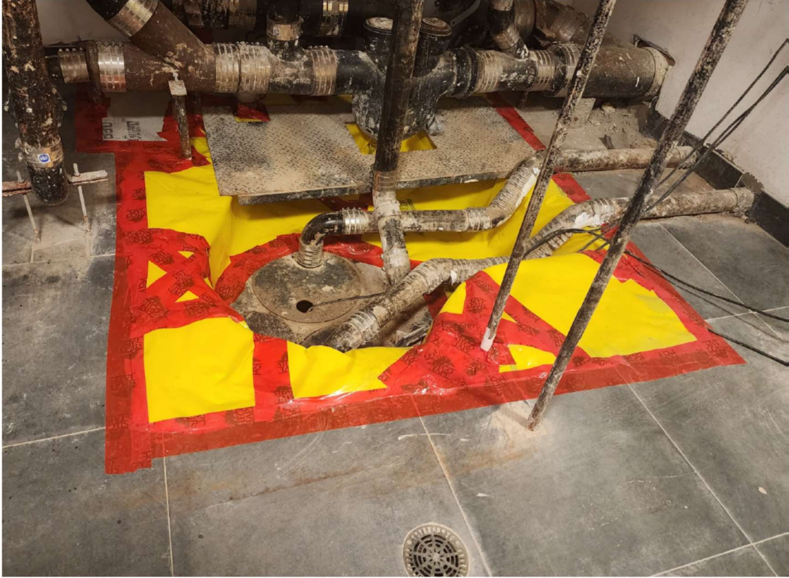
Photo 12 – View of Stego Wrap 20-Mil Vapor Barrier above the rubberized waterproofing extending over the tile, where vapor barrier remains under the tile in place.
