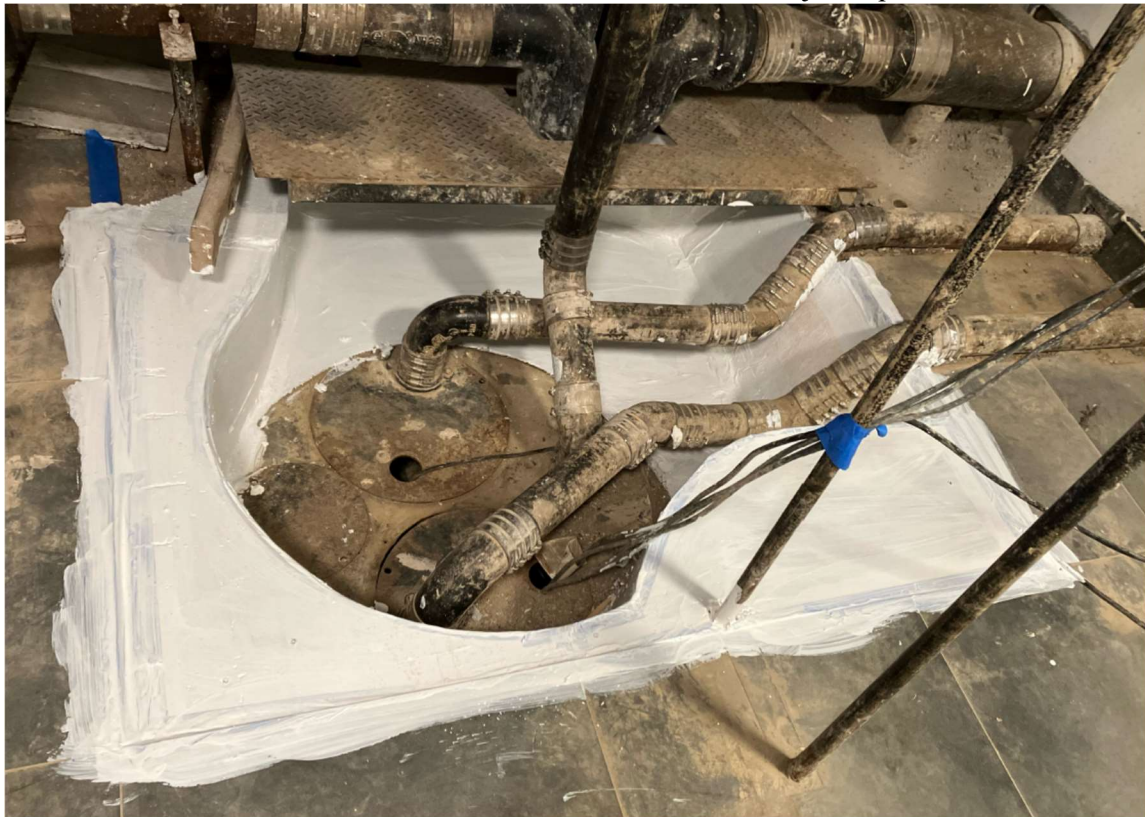
Photo 11 – View of Ames Rubberized Waterproofing applied around the form boards and over the floor in the area of the ejector pit.
