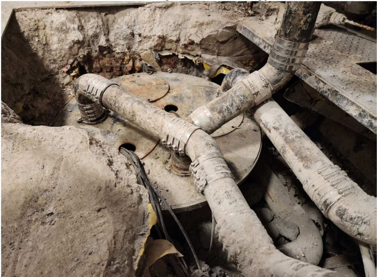
Photo 9 – View of ejector pit installation with vapor barrier voided during initial inspection in June 2023.
