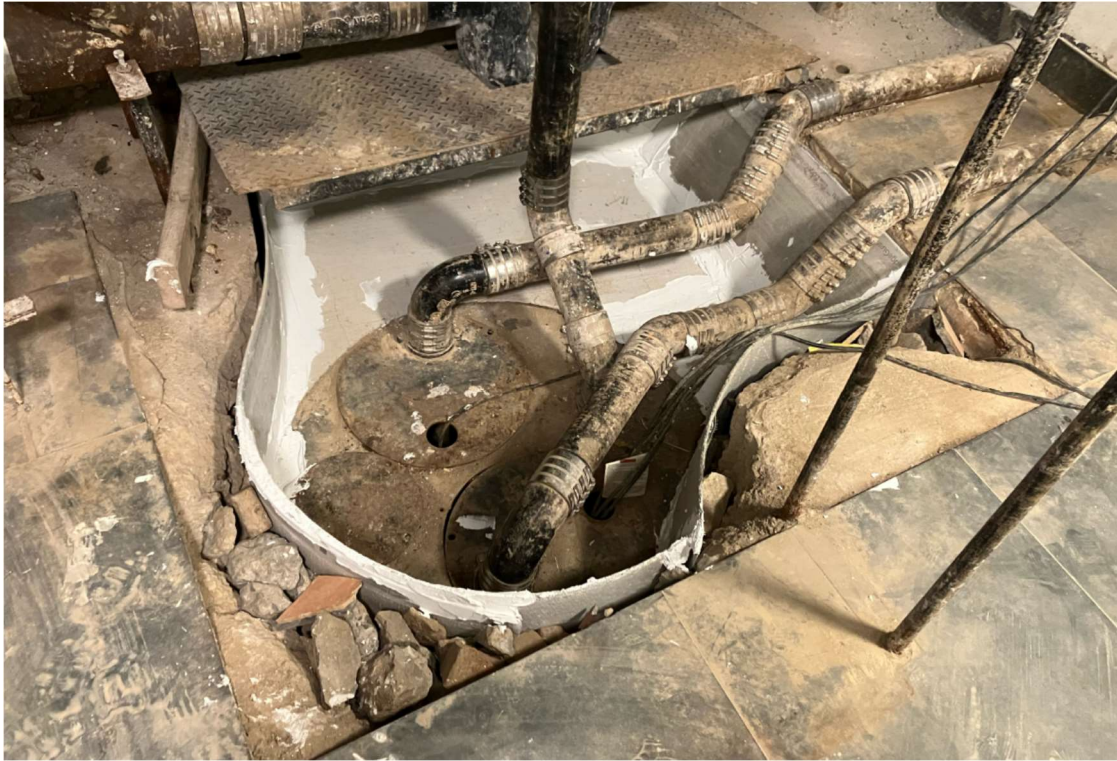
Photo 10 – View of form board installed around the ejector pit area.
