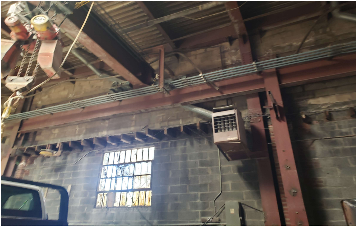
View of ceiling-mounted electric-fired space heater.
