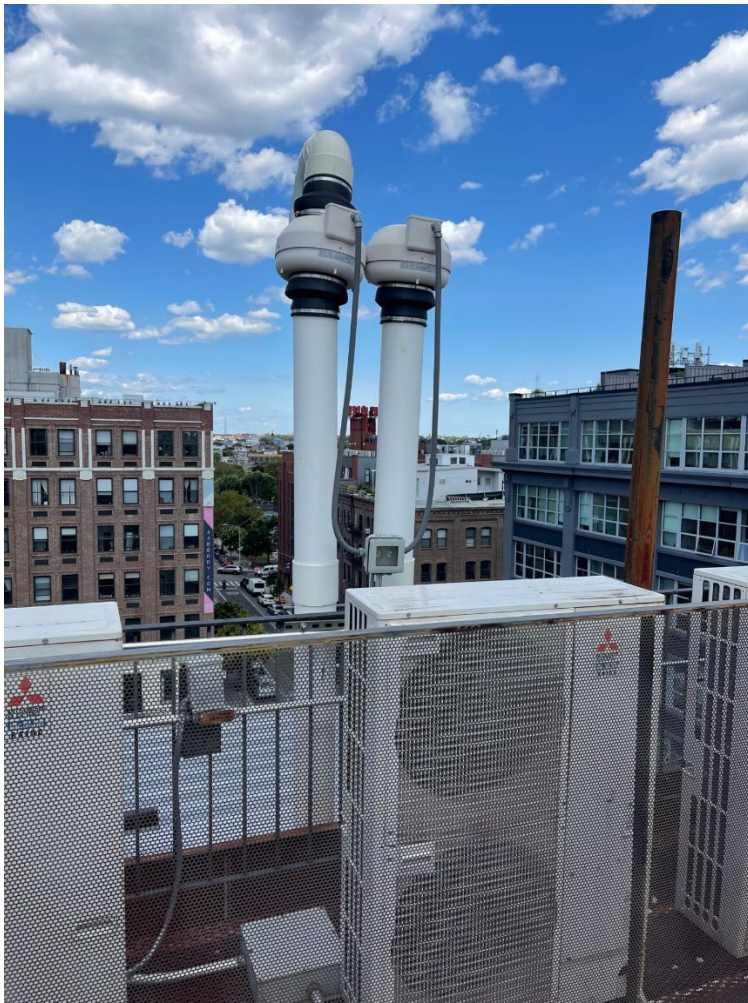
Photo 5. View of active SSDS risers/blowers installed on roof for cellar portion of building.
