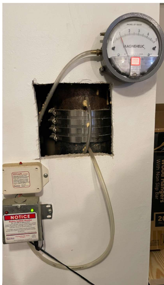
Photo 9 – View of the manometer and the alarm for the 237 Kent Avenue SSDS Loop.
