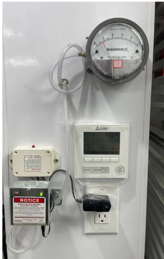
Photo 8 – View of manometer and alarm for the 235 Kent Avenue SSDS Loop.
