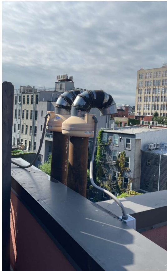
Photo 7 – View of blowers and risers on the roof of the 235-237 Kent Avenue
