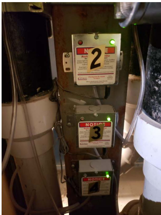
Photo 2: View of Riser 2, 3 and 4 alarms.
