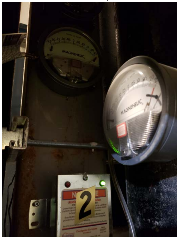
Photo 3 - View of Riser 3 and 4 gauges.
