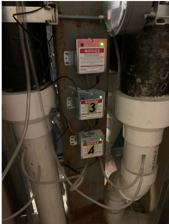
Photo 6 - View of replaced alarm for Riser 2.
