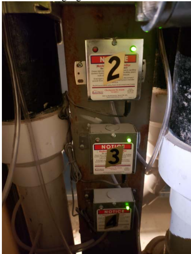
Photo 2: View of Riser 2, 3 and 4 alarms.
