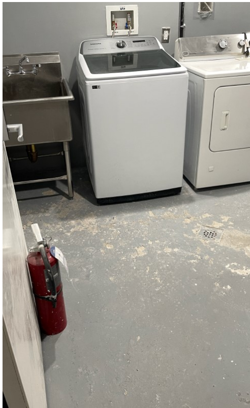
Photo 4: Additional view of cellar slab in the laundry room.
