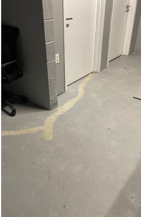
Photo 5: Additional view of the cellar slab.
