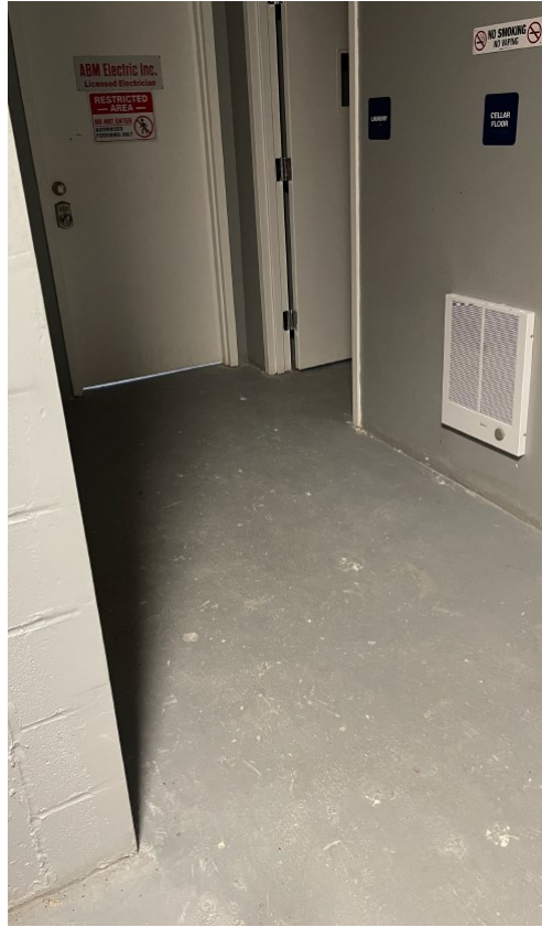
Photo 3: View of the cellar slab.
