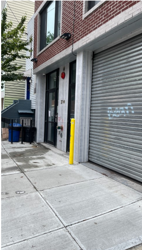
Photo 6: View of the front of the property along 39 th Avenue.
