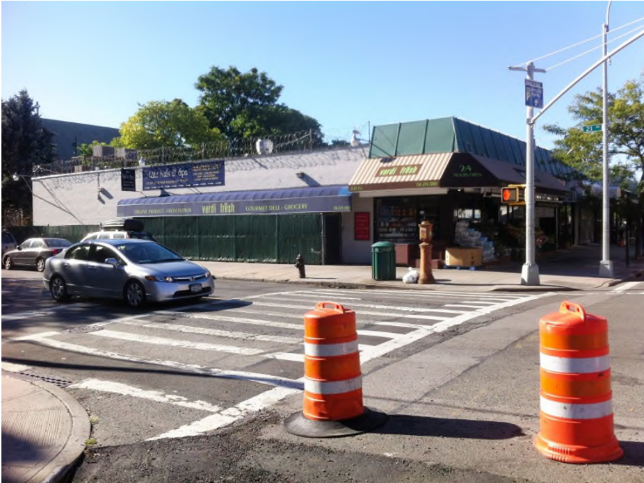
Photograph 1: View of the north section of the Site building looking south from across the intersection of 31 st Street and 21 st Avenue.
