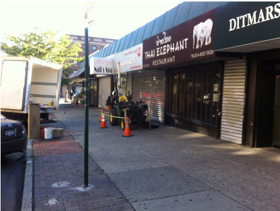
Photograph 2: Installation of Soil Boring B2. photographer looking north.
